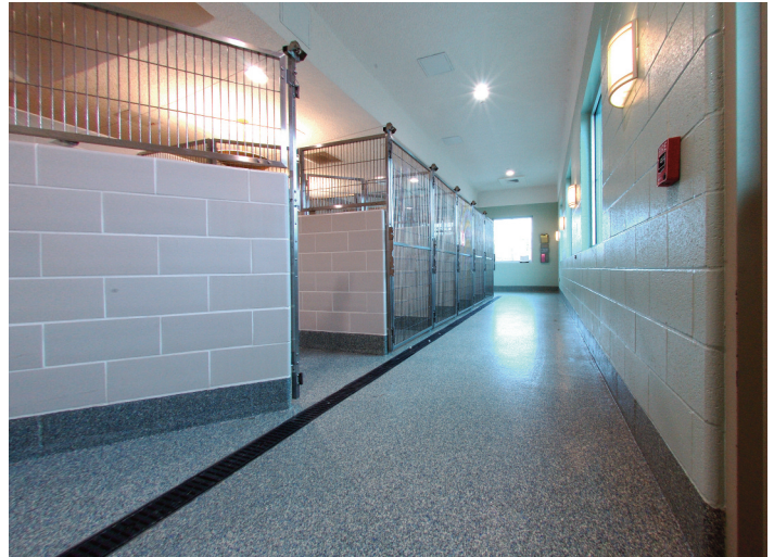
The wash down areas require slip-resistant, easy-to-maintain floors.
