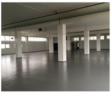
Stonclad GS, a troweled epoxy mortar system, provides this production facility with superior impact, abrasion and chemical resistance. Stonglaze VSR and VSD protect the walls from splashes, spills, fumes and abrasion.
