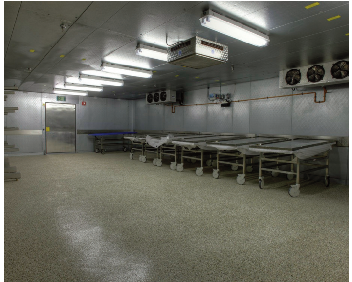
Stonhard's Stontec TRF and Stonblend GSI-G systems are hard-working, chemical-resistant, textured for slip-resistance and easy to clean at the District Nine Medical Examiner's Office.
