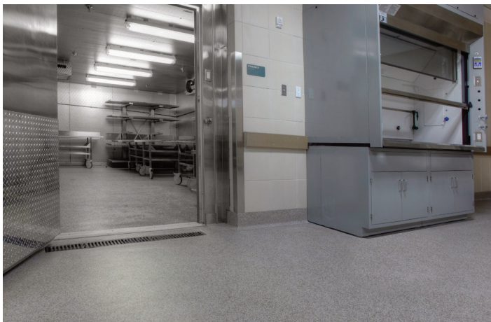
In the coolers, Stontec TRF floors are reliable, despite temperature extremes and heavy traffic.
